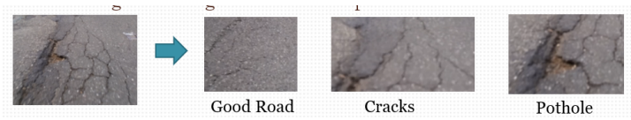
Fig. 17. Image showing both pothole and cracks, but was only labeled as 'cracks'
